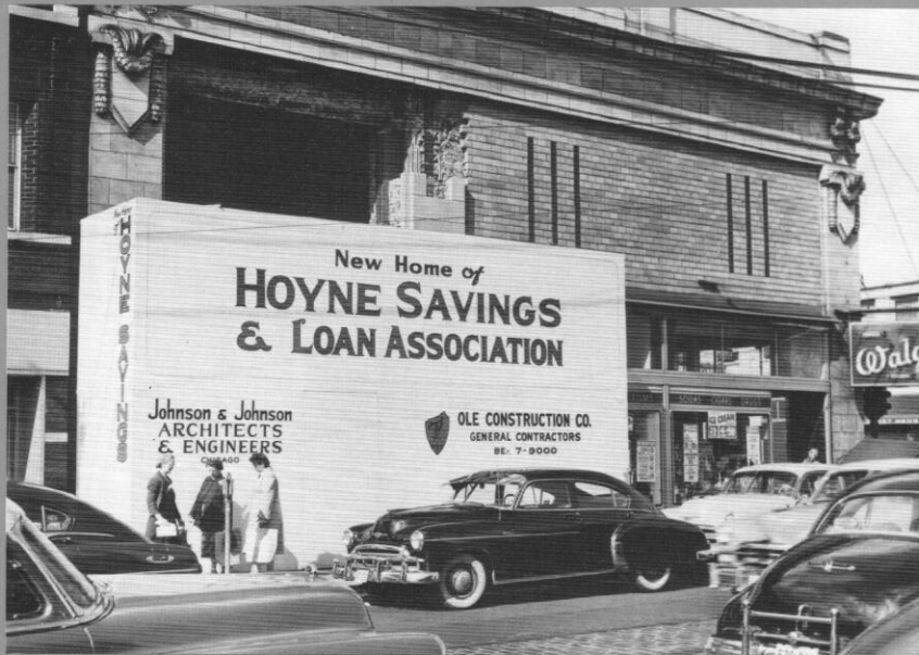
Hoyne's new main offices, undergoing extensive renovation, in 1954.
